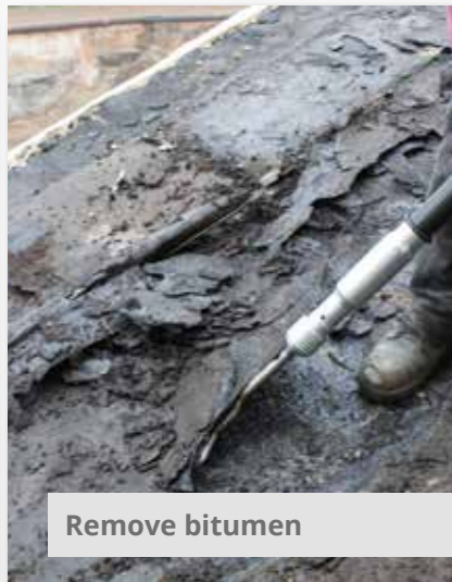
Pre-cutting bituminous sheeting
